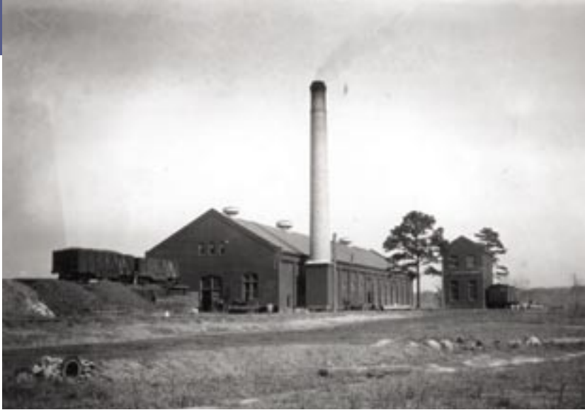
The original Hanahan Steam Pumping Station, pictured here in 1905. The building was refurbished in the 1980s and now houses the plant's administrative offices and laboratory.
