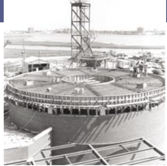
Construction of the Plum Island Wastewater Treatment Plant , 1968.
