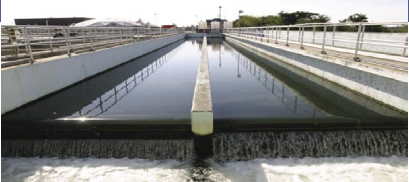
Wastewater effluent is disinfected in the chlorine contact tank before being released into the Charleston Harbor.
