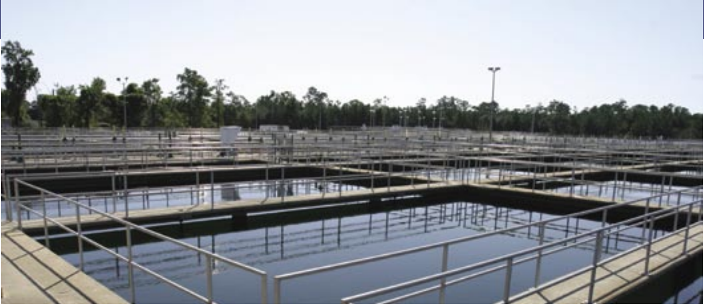
The sedimentation basins at CPW's Hanahan Water Treatment Plant.
