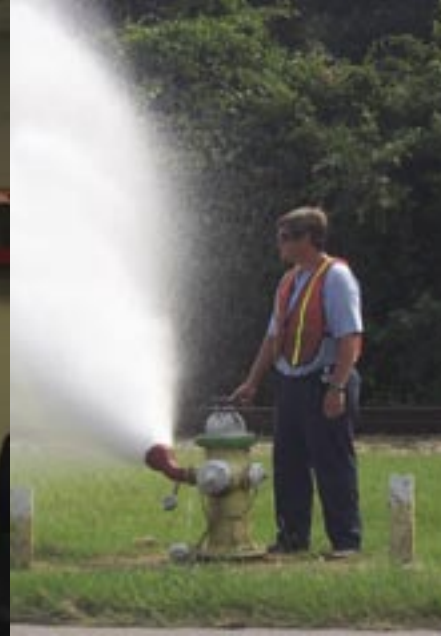
UDF Foreman Chris Dorn flushes a water main.
