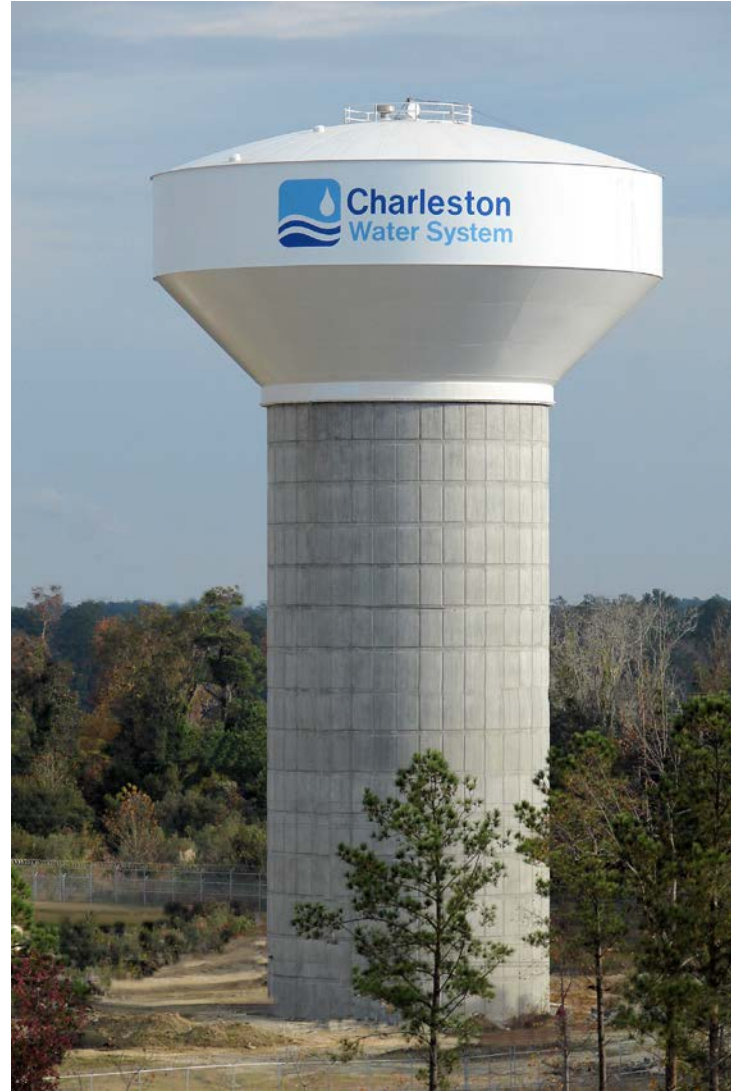
Located at the Hanahan Water Treatment Plant, the 1.5 million-gallon tank is Charleston Water System's newest elevated tank. It is used for backwashing and to maintain pressure in the distribution system in the event of loss of pumps.
