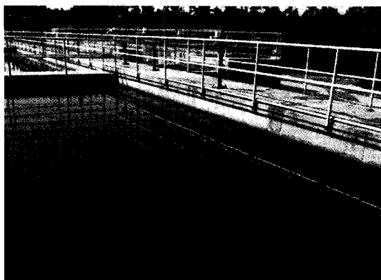
In this sedimentation basin, particles settle out of the water and are removed. The water then flows to the next step in the treatment process: filtration.
