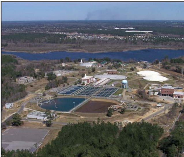
Hanahan Water Treatment Plant
