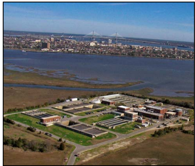
Plum Island Wastewater Treatment Plant
